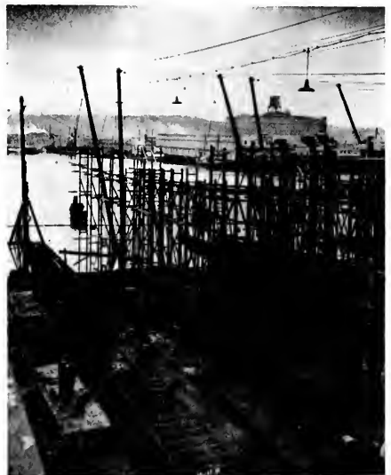
One of the ways at the Duthie yard, Seattle, showing inner bottom of one of the big freighters building at this plant.
